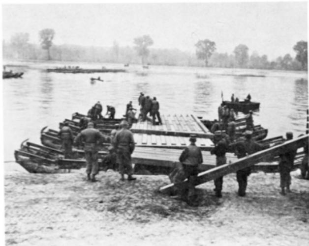
Aluminum baulk being installed
