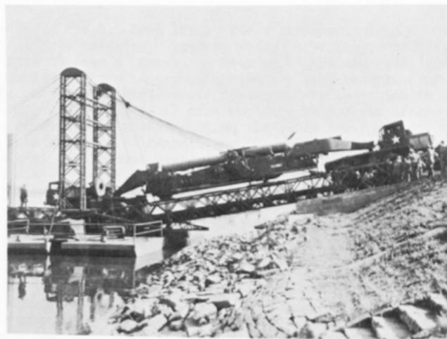
Ramp section w/Ramp tower assembly
